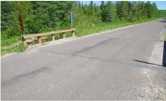
Deterioration at Guide Rail Attachment
