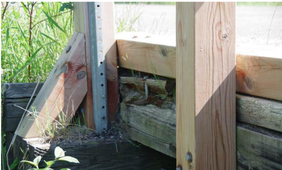
Deterioration at Guide Rail Attachment
